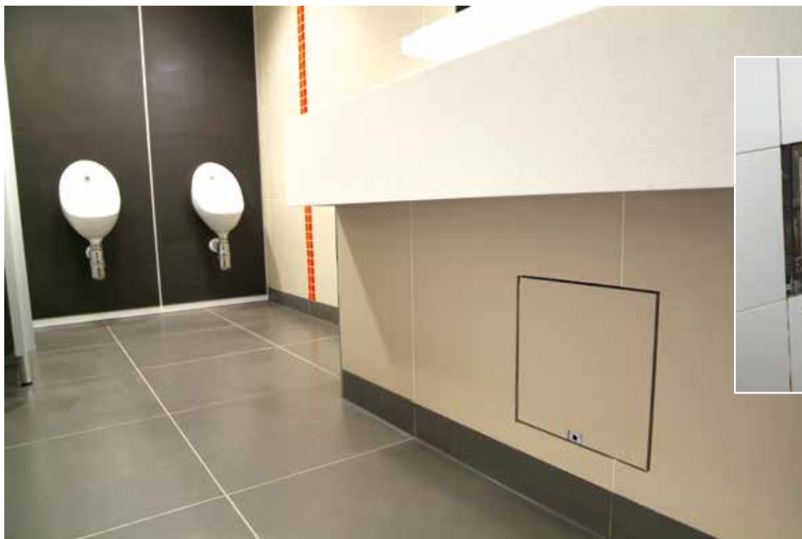
Main image (left) shows security locking system, inset (above) shows concealed push/pull locking mechanism
