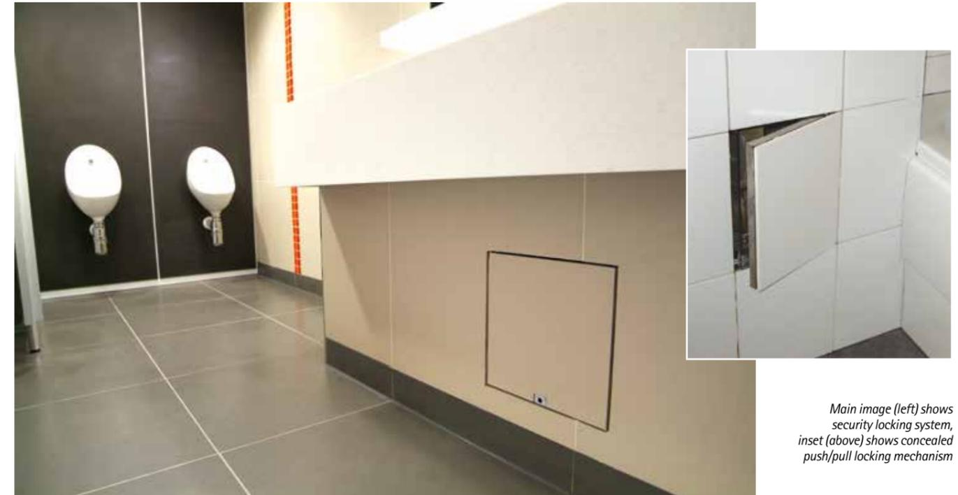
Main image (left) shows security locking system, inset (above) shows concealed push/pull locking mechanism
