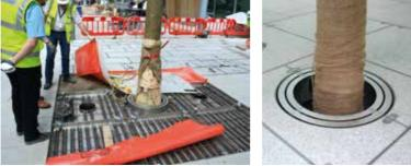
Top: Tree Pit cover in an indoor environment Bottom left: Typical construction process for Tree Pit covers Bottom right: Tree Pit cover in an outdoor environment
