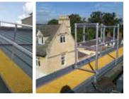
1. Pedestal For gutter cleaning access.
