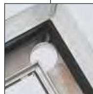
Top-side - Water drainage channel with drainage outlet
