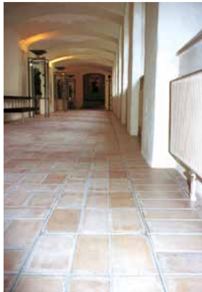
Filled with tiles - continuous run of covers through length of corridor
